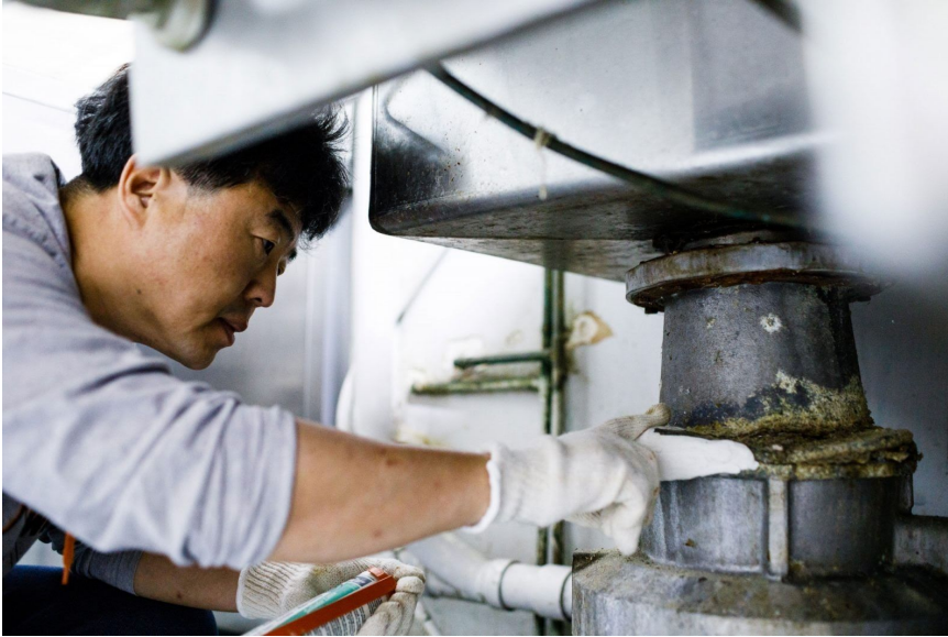
Yeom makes some repairs as he prepares for a health inspection for his new restaurant. Yeom bought a fish market after working in the chicken plant for 13 months.
